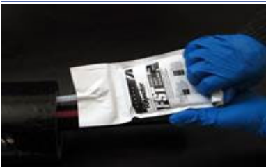
Injection du FST Burst Pack.
