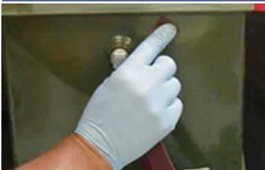
Sand or brush repair area
