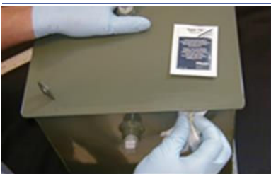
Clean area with cleaning wipe before applying sealant
