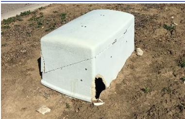
Large holes need backing
