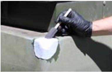
Attaching fabric to enclosure
