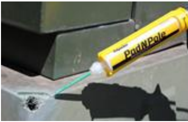
Applying thin coat of Pad N Pole
