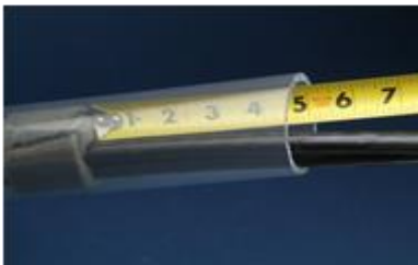
Measure foam dam depth.
