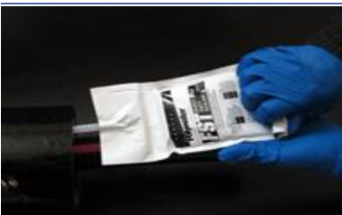
Injecting FST Burst Pack.
