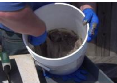
Mix the Sika colorant into the blend
