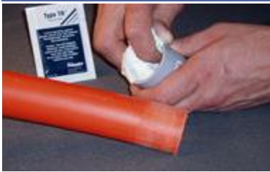
Clean Coupling and Conduit with Cleaning Wipe
