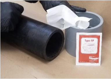
Clean Coupling and Conduit with Cleaning Wipe
